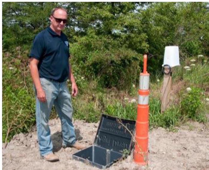
Kyle VanTilburg at the controlled drainage structure. Stop logs are controlled within this control box to allow the rise and fall of the water table with the tile lines, allowing plants to absorb more water.
